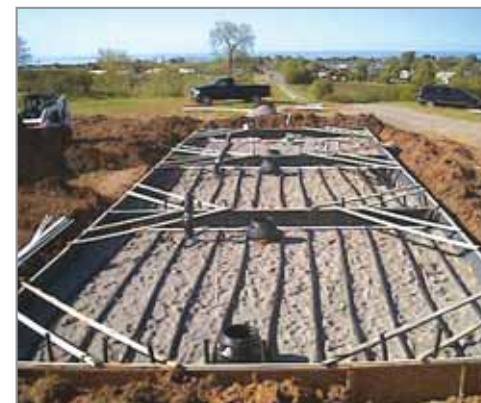
Left: A three-cell vertical wetland under construction, including pump chambers, perforated collection pipes and a 30-mil PVC liner that is flexible for easy installation and pliable in cold weather. Center: The vertical wetland components are covered with filtering media, which varies depending on treatment objectives and wastewater characteristics (i.e., particle size, porosity and aluminum, iron and calcium content) and treatment objectives. Right: The vertical wetland is planted with cattails (Typha sp.) or reed grass (Phragmites sp.), again depending on wastewater characteristics (Phragmites, for example are more tolerant of high ammonia concentrations).
