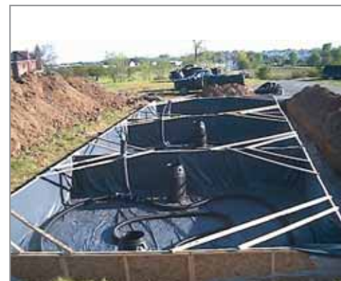
Left: A three-cell vertical wetland under construction, including pump chambers, perforated collection pipes and a 30-mil PVC liner that is flexible for easy installation and pliable in cold weather. Center: The vertical wetland components are covered with filtering media, which varies depending on treatment objectives and wastewater characteristics (i.e., particle size, porosity and aluminum, iron and calcium content) and treatment objectives. Right: The vertical wetland is planted with cattails (Typha sp.) or reed grass (Phragmites sp.), again depending on wastewater characteristics (Phragmites, for example are more tolerant of high ammonia concentrations).
